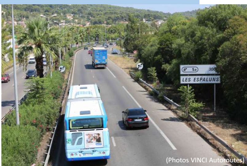
(Photos VINCI Autoroutes)
